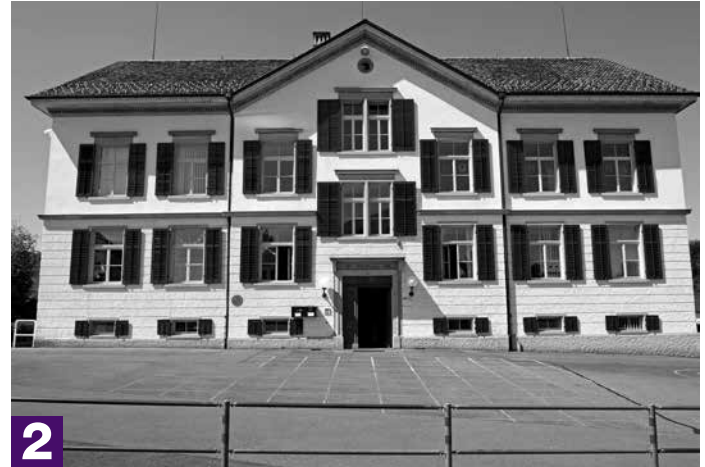
2 Schulhaus Dörfli, Oetwil am See, 1889
